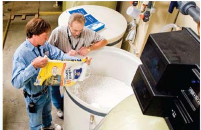
**PHOTO:** Boeing heating, ventilation and air-conditioning mechanic Brett Weberg adds salt used in regeneration tank for cooling-tower water softeners at the Kent, Wash., site. The water softener is part of a new process initiated by lead mechanical engineer Roger Sampair (right) that will save water and reduce sewage and maintenance costs across Boeing. **MARIAN LOCKHART/BOEING**
